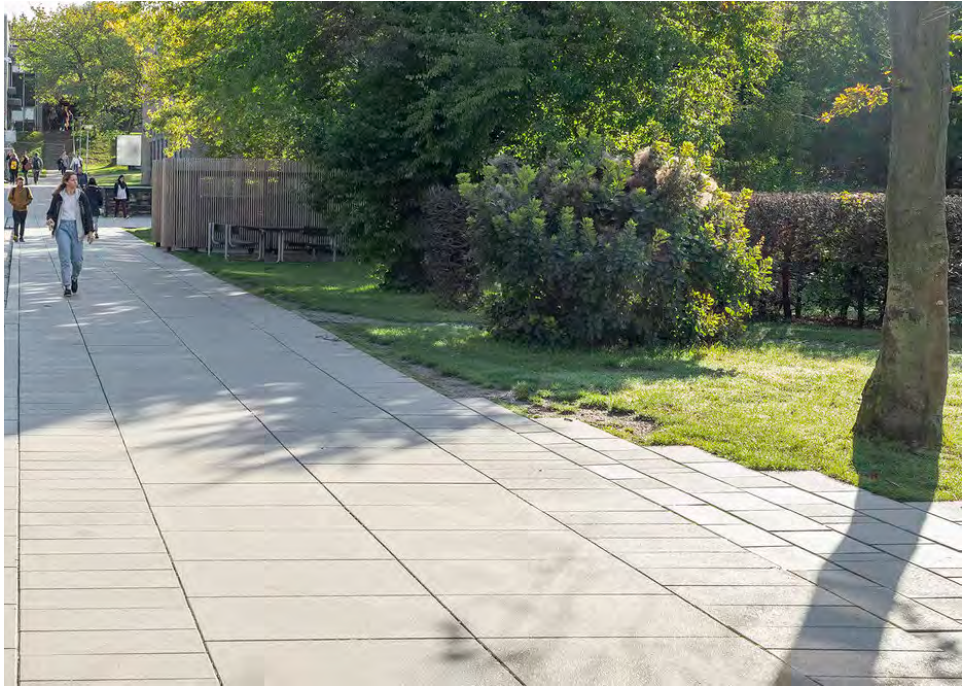
betontegels 50x50 cm in blokverband
